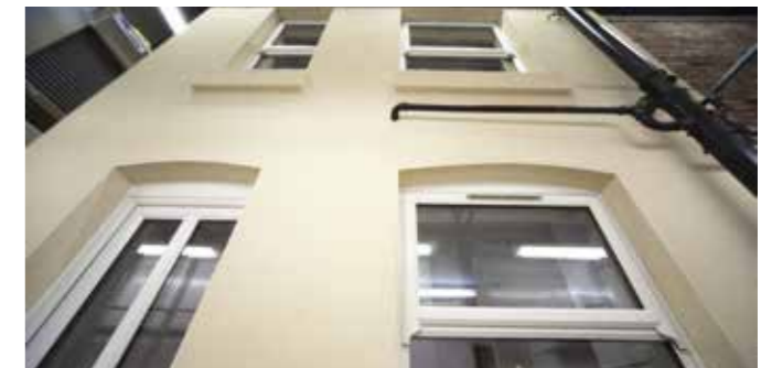
Rear elevation, with external wall insulation
