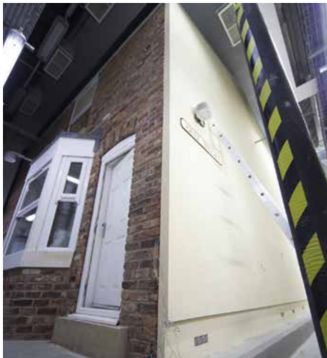
External wall insulation to gable
