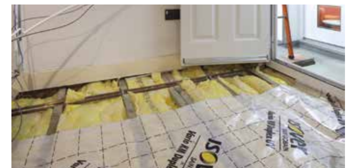
Floor insulation installation with vapour permeable membrane
