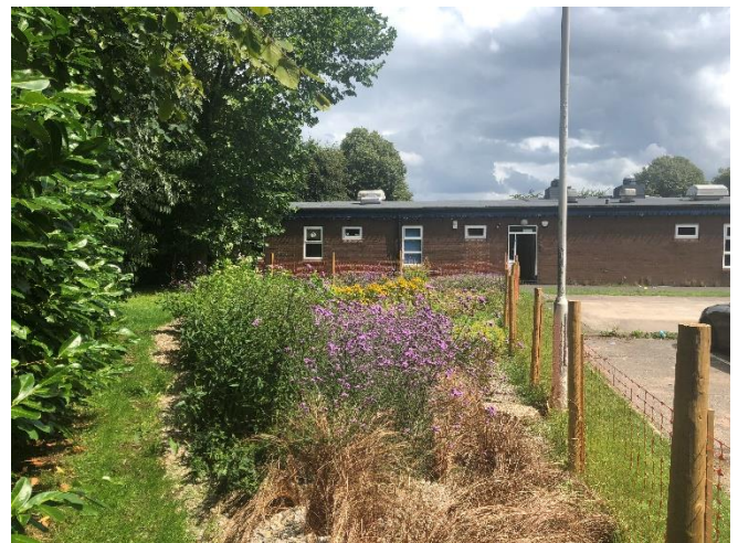
Shaw Heath NHS Health Centre, Rain Garden A pilot site for the Water Resilient Cities work
