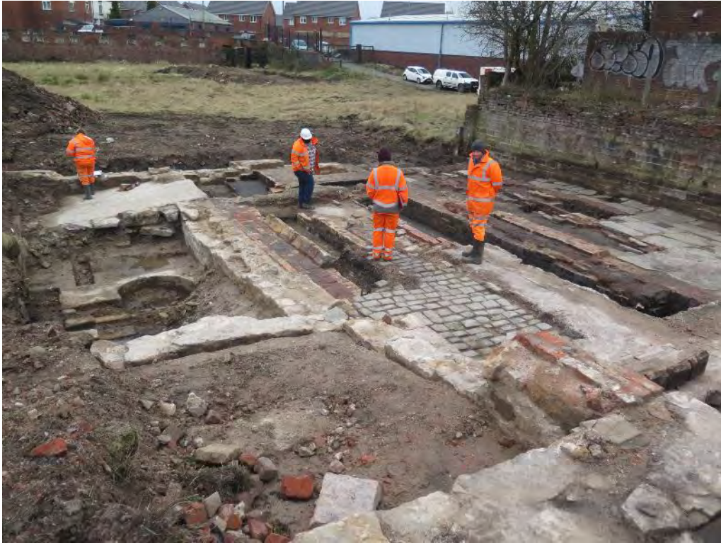
Victoria Mill excavation. The former canal arm site is just beyond the figures. A granite sett surface in the centre of the photo is a late 19 th century phase overlying remains of an early boiler and in turn overlaid by a 20 th century concrete slab. The engine house remains are on the left, flanked by solid stone wall.
