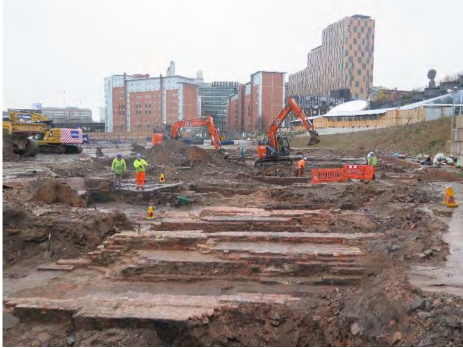
Excavating the site of Hoyle's Print and Dye Works, with a series of boiler beds evident in the foreground and the former Mayfield Railway Station to the upper right of the picture
