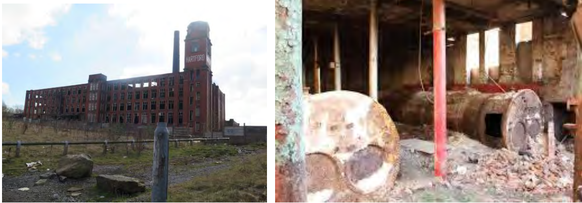
Hartford Mill: view showing poor condition of the mill (left) and the boiler house (right)
