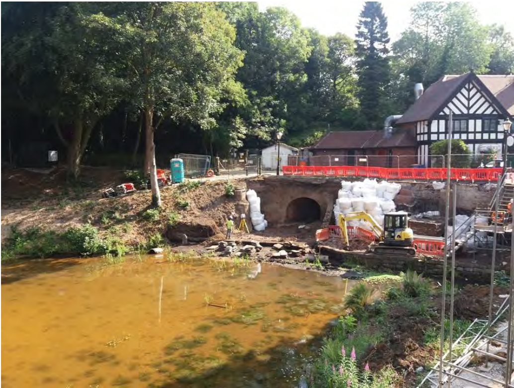
Worsley Delph showing the previously unknown tunnel entrance and stone quayside exposed and recorded during ground works
