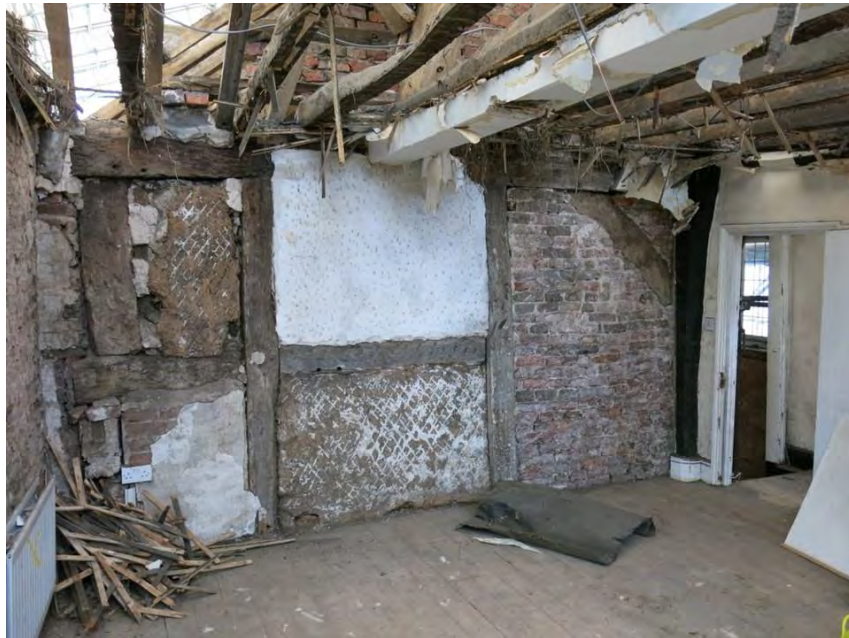
Woodford Old Hall showing internal timber framing and infill panels, revealed during the soft strip
