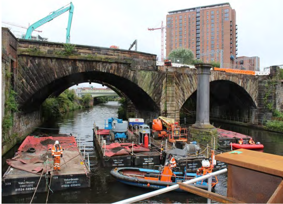
Ordsall Chord: the 1830 Stephenson Railway Bridge after removal of the Girder Bridge
