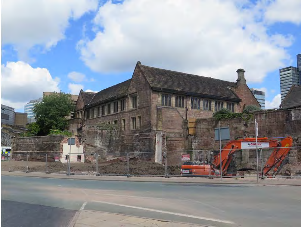
Removal of the Palatine Building has revealed the late medieval precinct wall and bedrock beneath Chetham's College. The rocky outcrop was the site of Manchester Castle.
