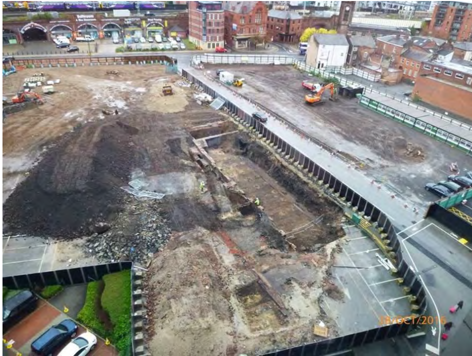
Chapel Wharf Phase 3 development site, viewed from the Lowry Hotel, showing the basement of Salford Twist Mill which retained archaeological evidence for world leading textile mill technology
