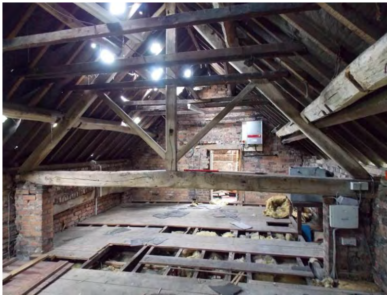
The 18 th century timber roof structure
