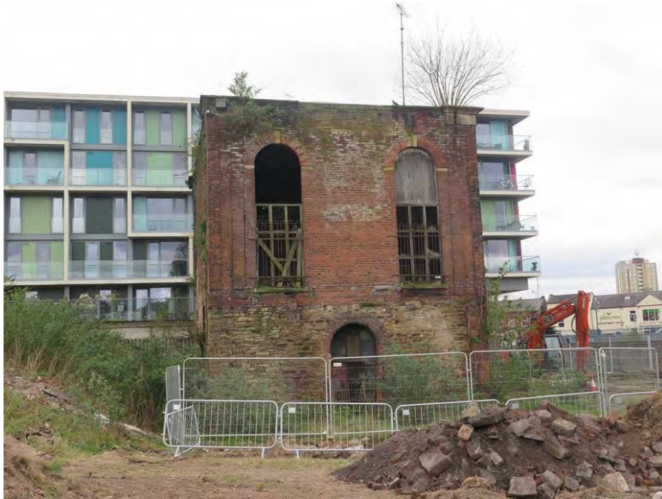
Castle Street Mill, Stalybridge. Remains of the detached (listed) engine house with archaeological evaluation trenching taking place
