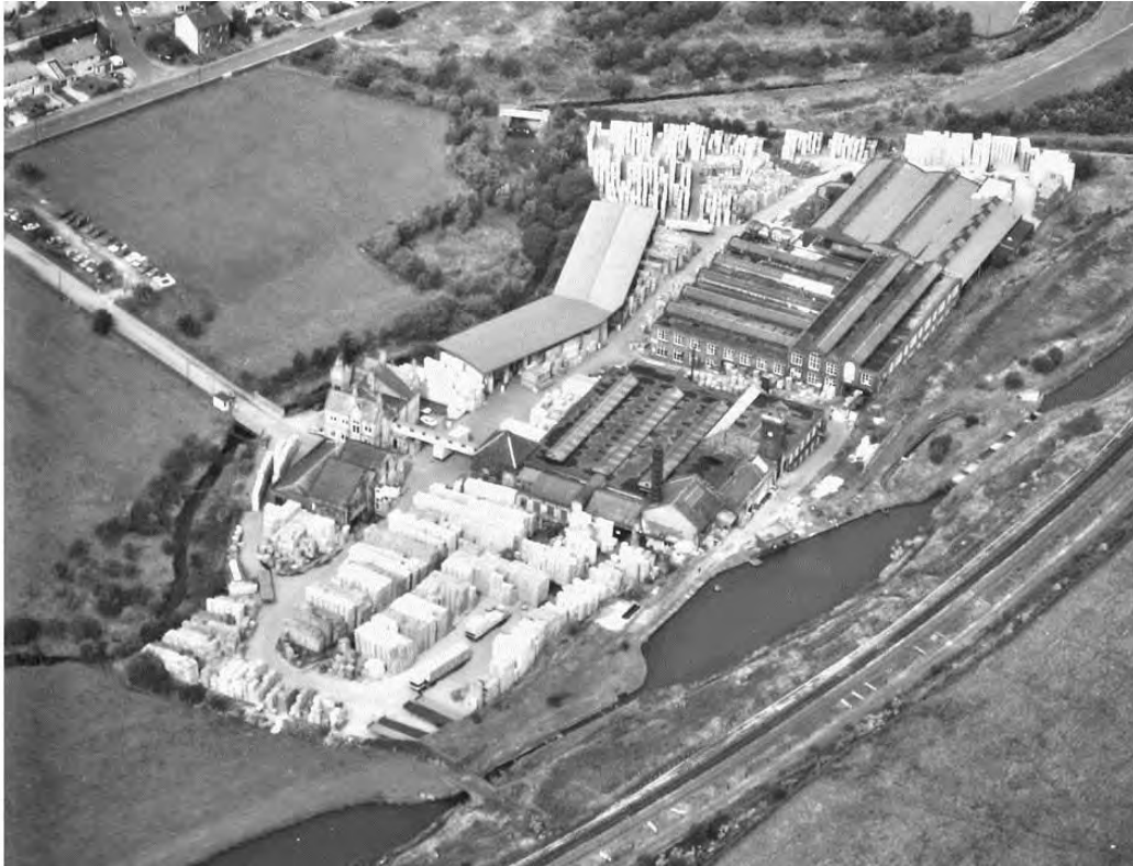
Oblique aerial view of Dobcross Loom Works in the late 1980s (source: GM Textile Mills Survey)
