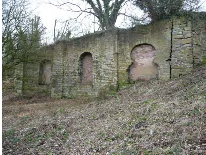
The remains of Oldknow's lime kilns in Marple
