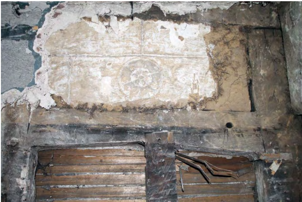
Kempnough Hall: Removal of plaster reveals original timber framing and plaster 'rose' motif above former doorway
