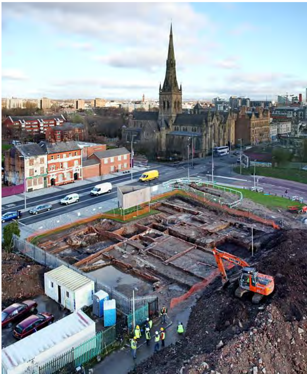
Chapel Street open area excavation
